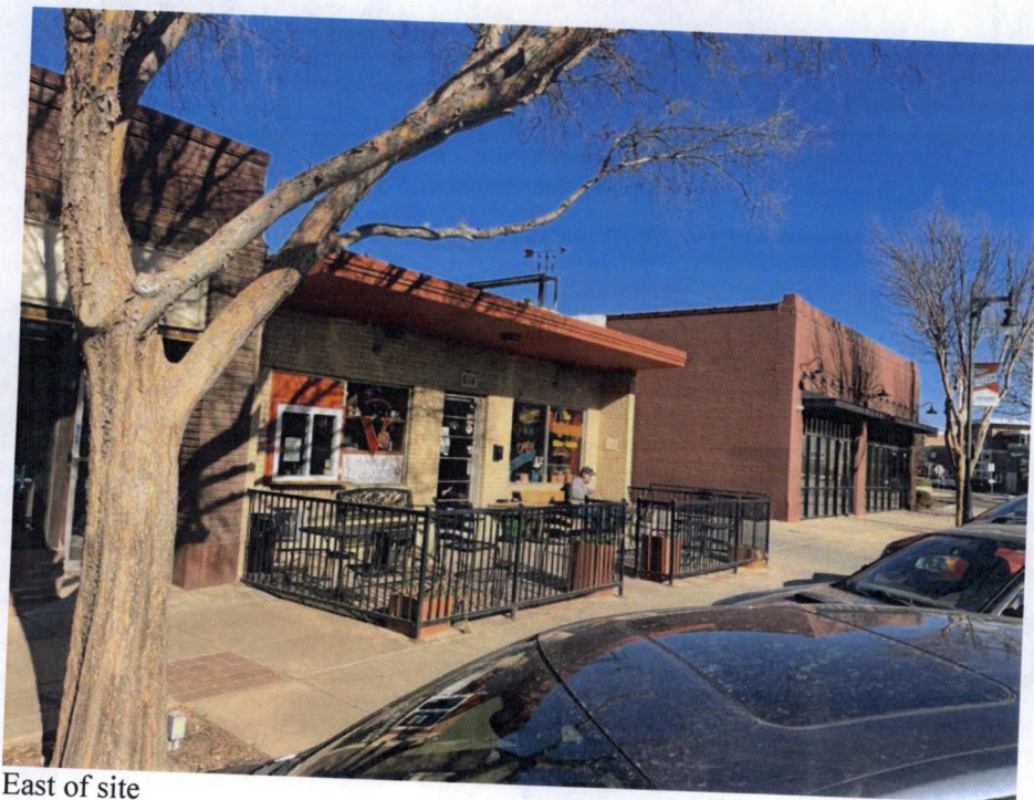
Site looking north
