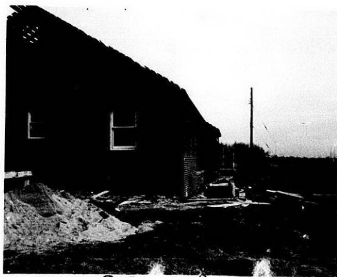
5502 E. Pine - Looking NE.
