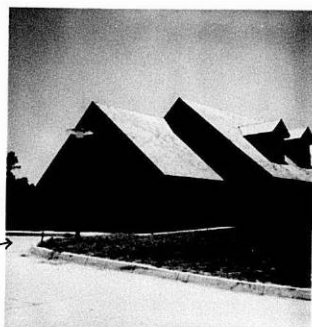
Someone leaving the front entrance would have to pass brick wall to get to parking
