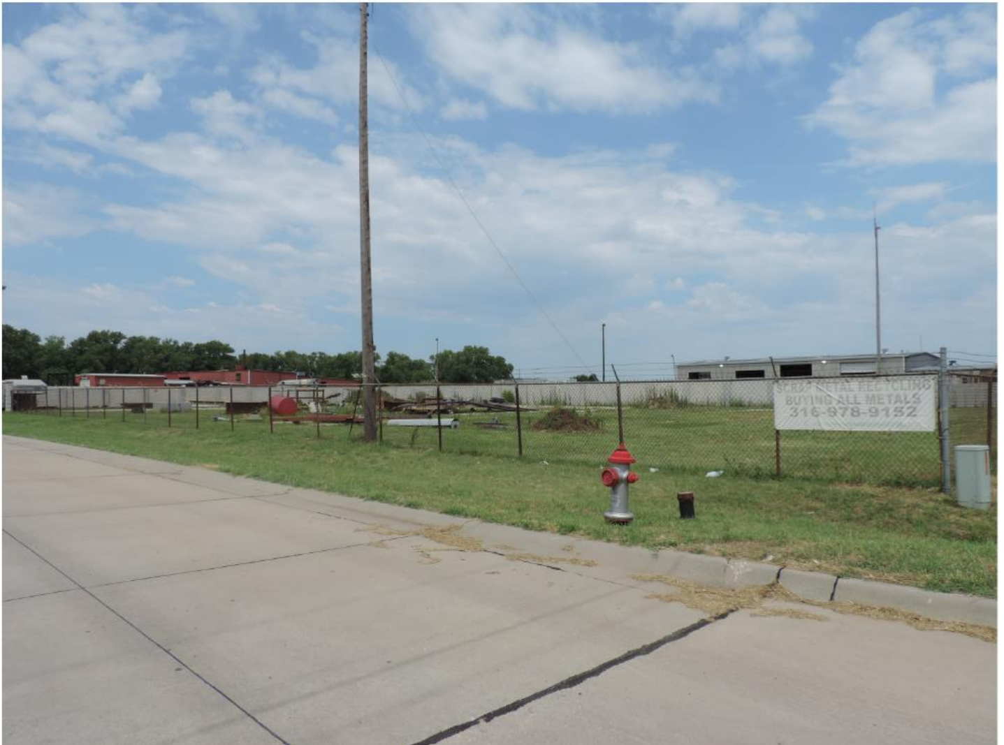
Site looking north with utilities in South Hoover Ct ROW
