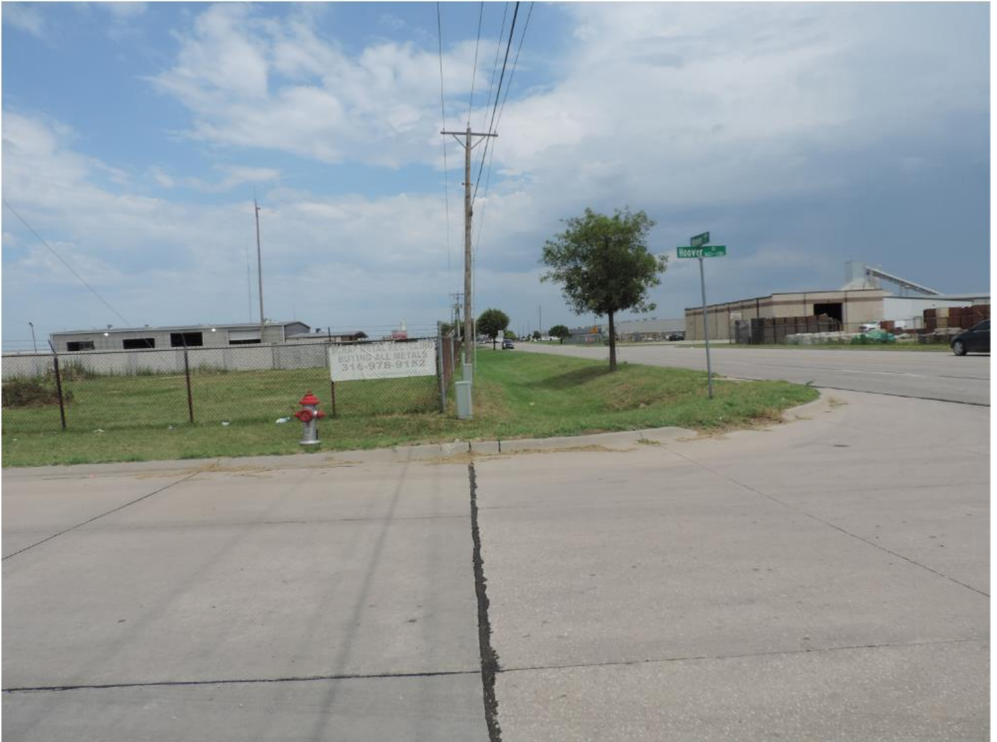
Site looking north with utilities in South Hoover Rd ROW
