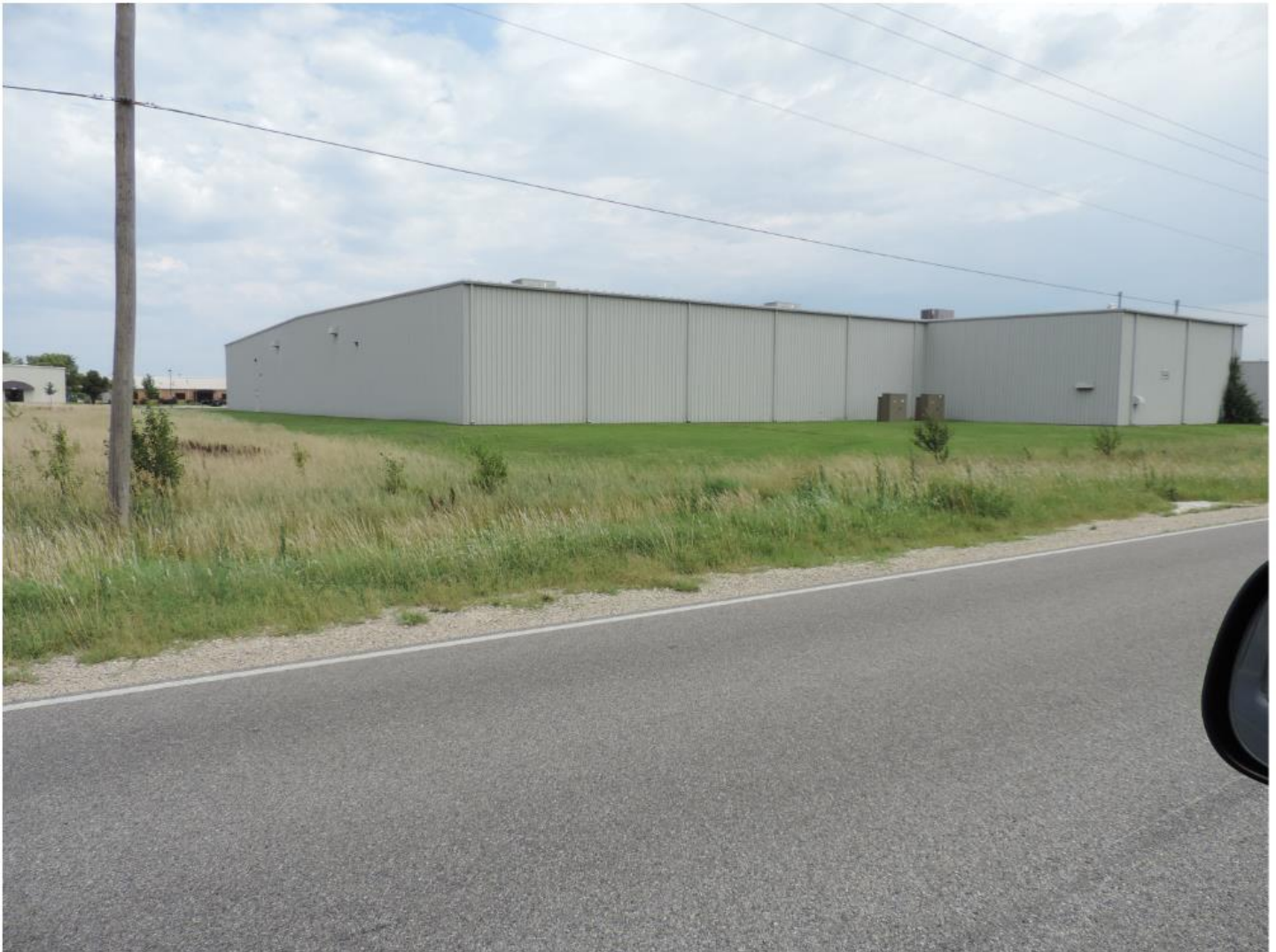
Site off of West MacArthur Rd where expansion and proposed driveway will be located
