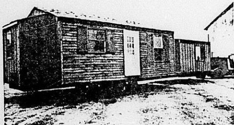
Echo house in transit.
