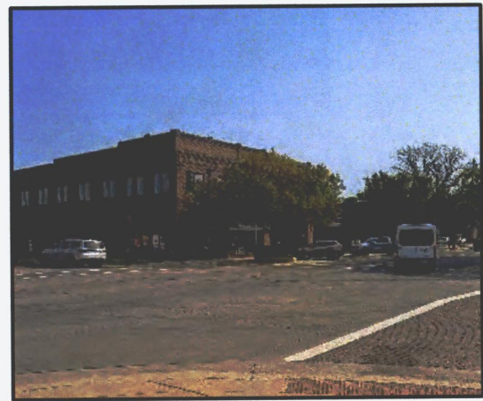
Northeast corner of Handley & Douglas - BBQ shop
