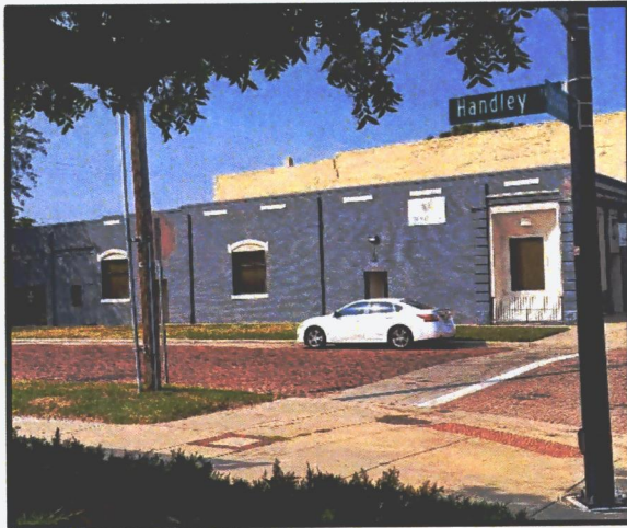
East side of building at 901 W. Douglas
