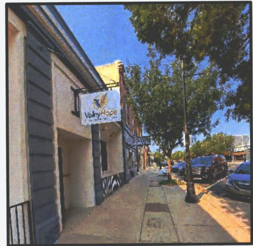
Front of 901 W. Douglas and viewing west
