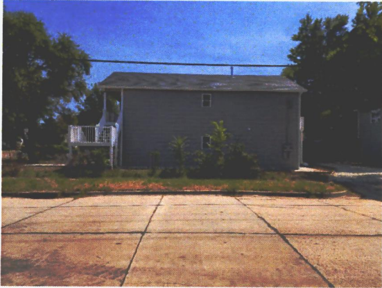
Looking south towards main structure
