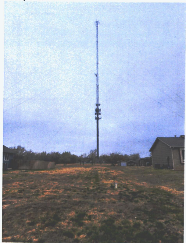
Looking northwest towards existing telecommunications tower on Winesap Street
