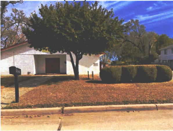
Looking east at church property
