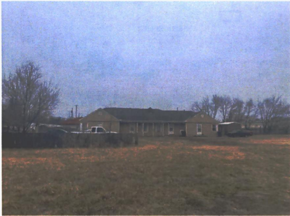
South of the subject site.
