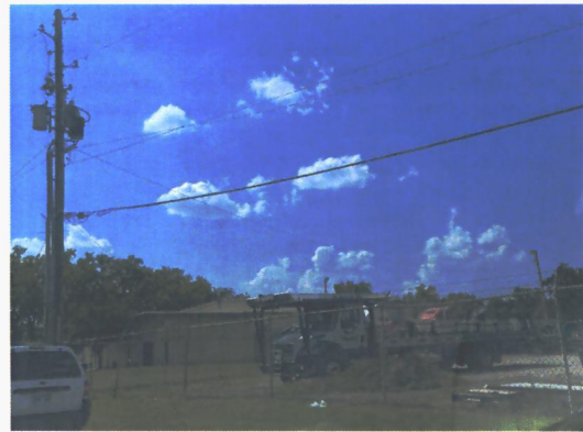
South side of subject site.
