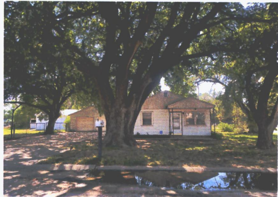
Single-family residence north of subject site.
