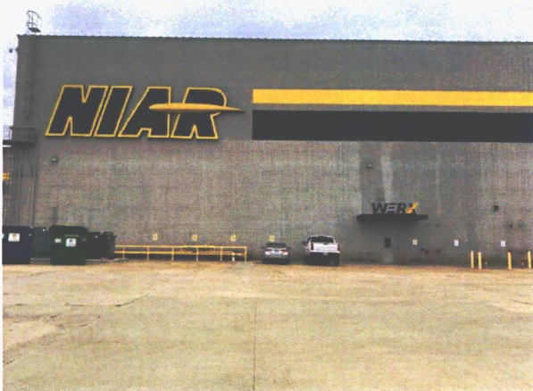
Looking east towards existing sign
