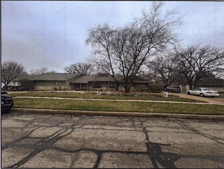
Looking west into site
