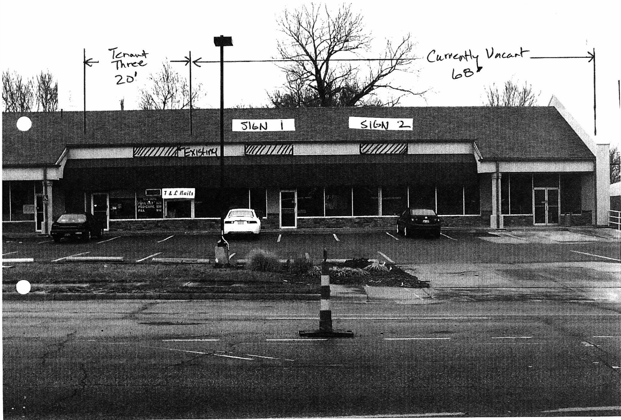
EAST END OF SHOPPING Center
