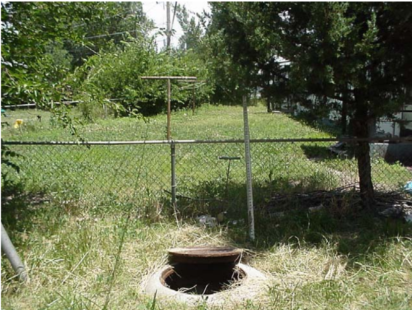
Standing west of MH 5744-694, looking east.
