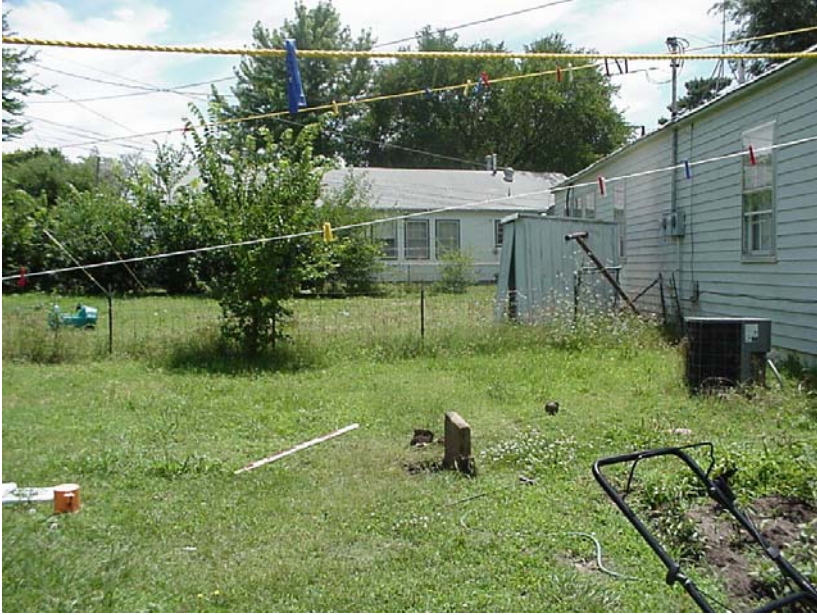
Standing north of Cleanout 5744-697CO, looking southerly toward MH 5744-693. There is a concrete block over the cleanout (block is standing on-end in the picture).
