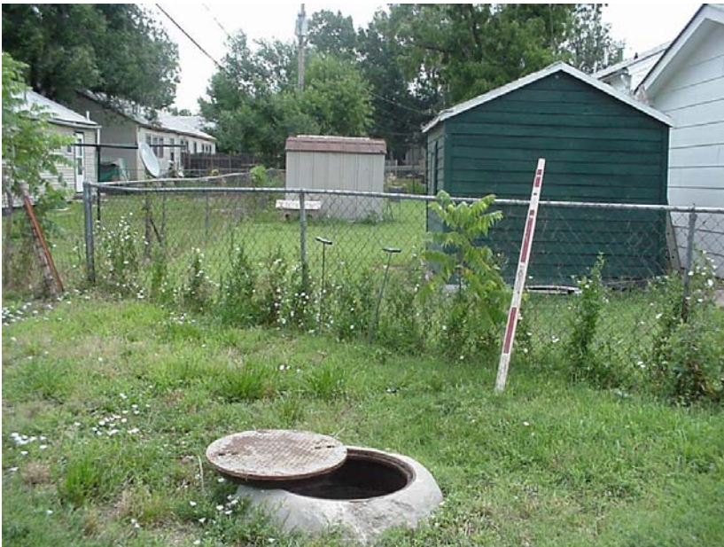
I'm standing west of MH 5744-689, looking east.
