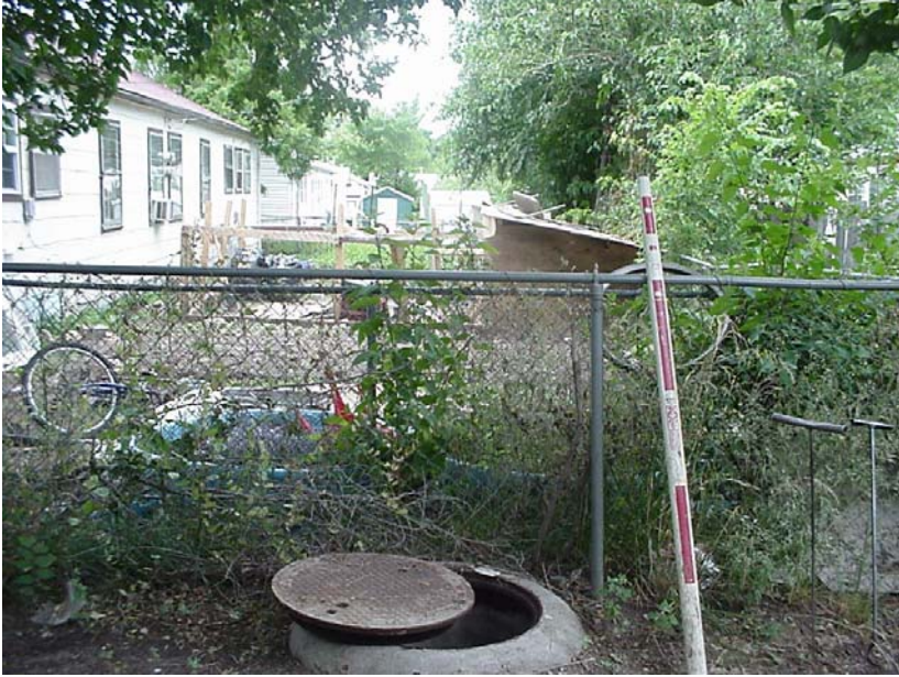
I'm standing east of MH 5744-690, looking west.
