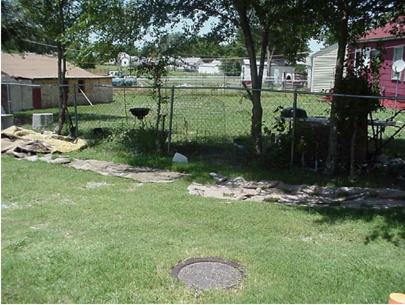
Standing southeast of MH 5744-717, looking northwest
