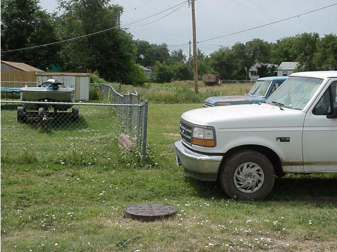
Standing north of MH 5744-686, looking south.
