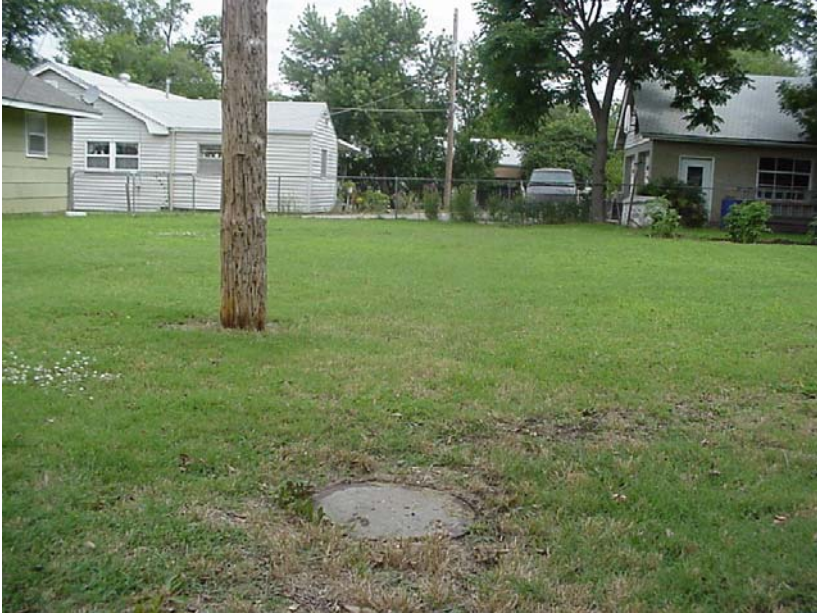
Standing south of MH 5744-699, looking north.
