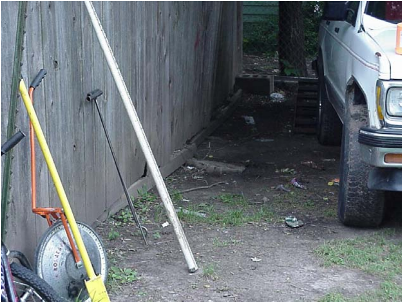
Standing north of Cleanout 5744-701CO, looking south. In the yard of 3426 E. Dunham, on the west side of the wood fence under a concrete patio block.
