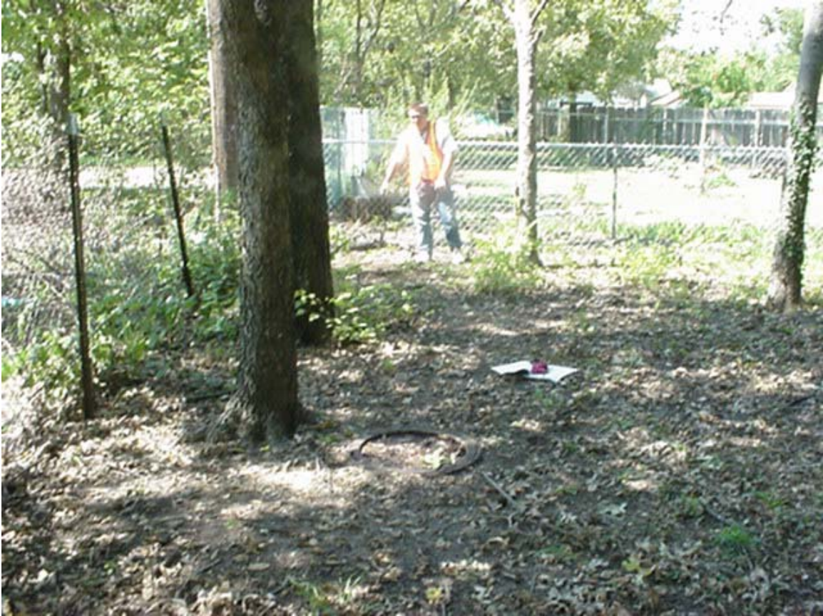
Two manholes in the yard of 319 N. Athenian. MH 5347-567 is in the foreground at the base of the first tree. MH 5347-xxx (to be abandoned) is closer to the fence, where Greg is standing.
