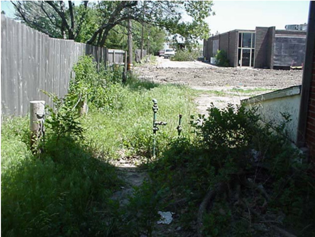
Standing at the east edge of 8302 E. Kellogg, looking east toward vacated Bonnie Brae. There are two vertical gas pipes that are blocking the entrance to the easement. Contractor is responsible to make the necessary arrangements for access to the easement.
