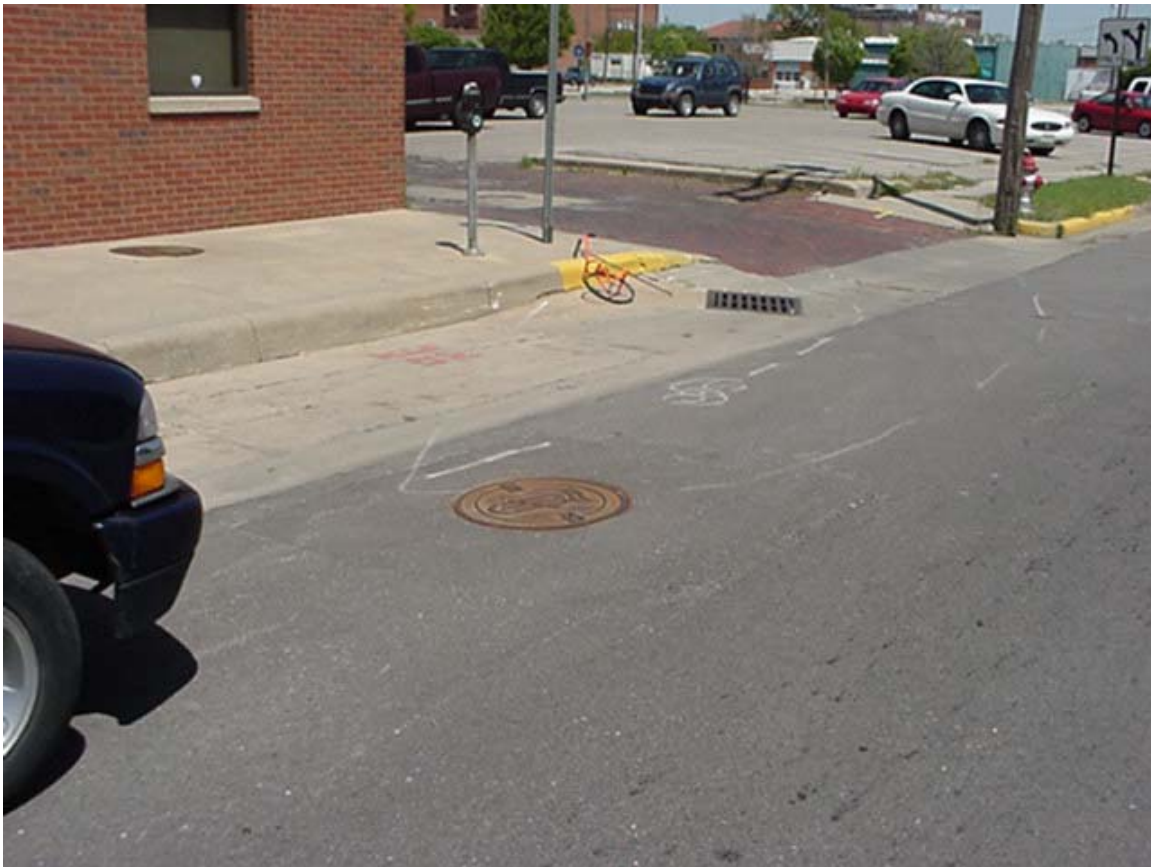
Standing SW of MH 5547-041, looking NE
