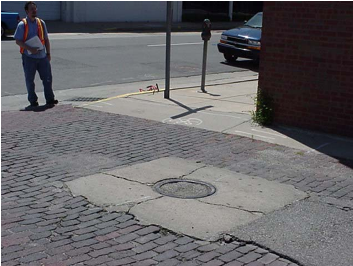
Standing NE of MH 5547-042, looking southwest. A straight line to MH 5547-041 would put the pipe between the sign post and the parking meter.
