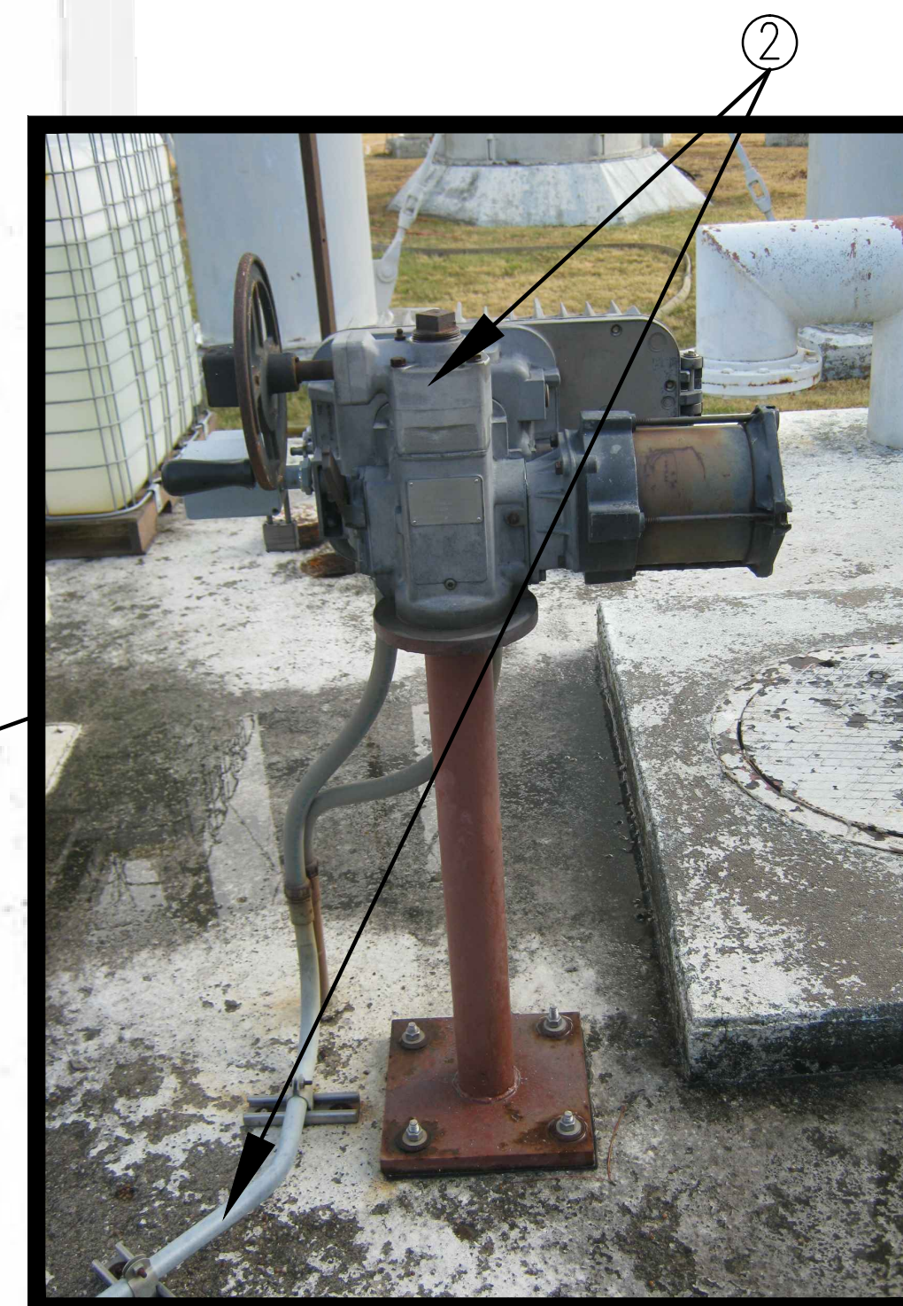
ELECTRIC BUTTERFLY VALVE ACTUATOR
