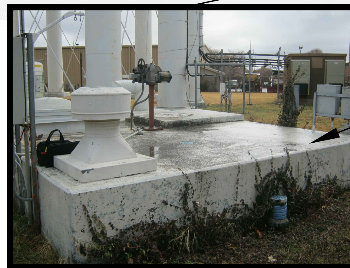
TOP OF VAULT VIEW
