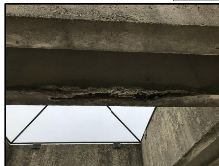
EXISTING CONCRETE STRUCTURE
