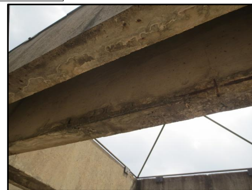
EXISTING CONCRETE STRUCTURE
