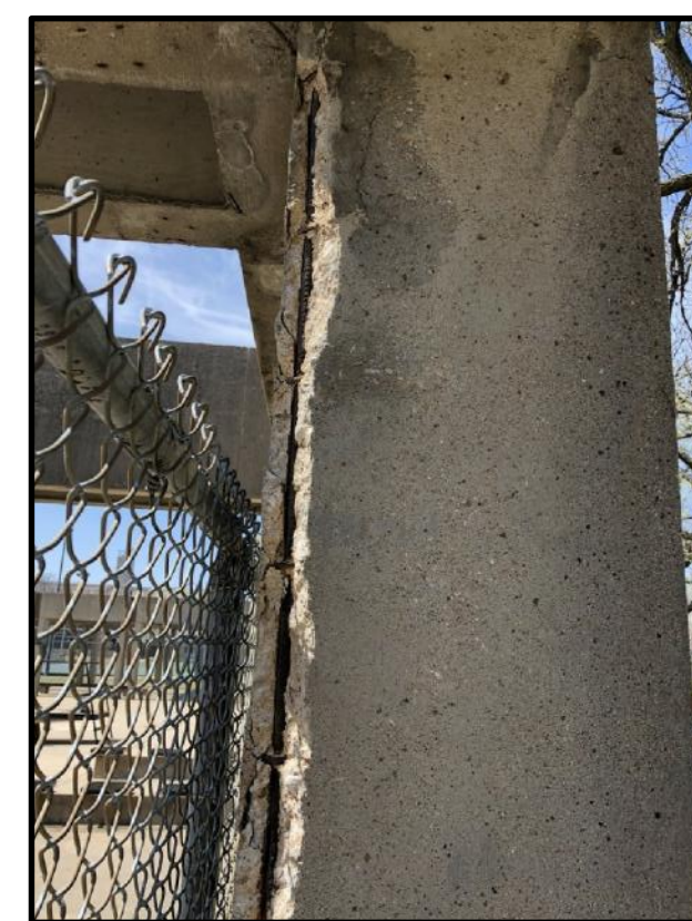
EXISTING CONCRETE STRUCTURE
