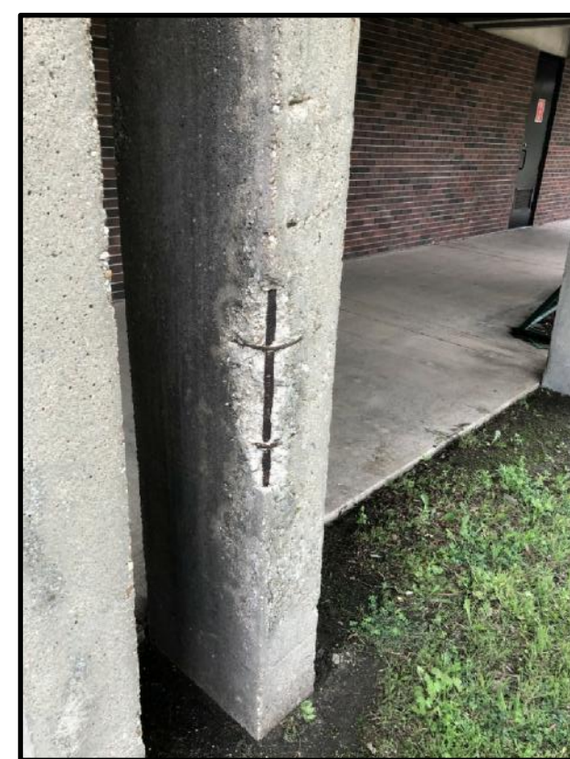
EXISTING CONCRETE STRUCTURE
