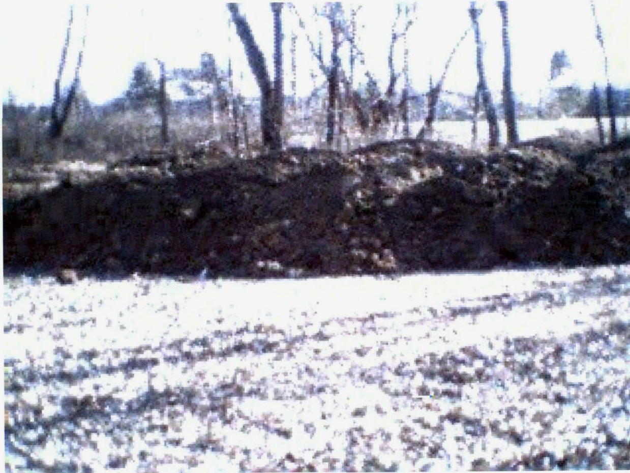
DIRT PILE LOOKING TOWARD CLOISTERS DRIVE
