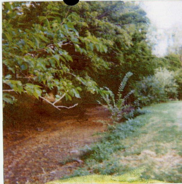
2. VIEW OF POND OUTLET CHANNEL LOOKING UPSTREAM
