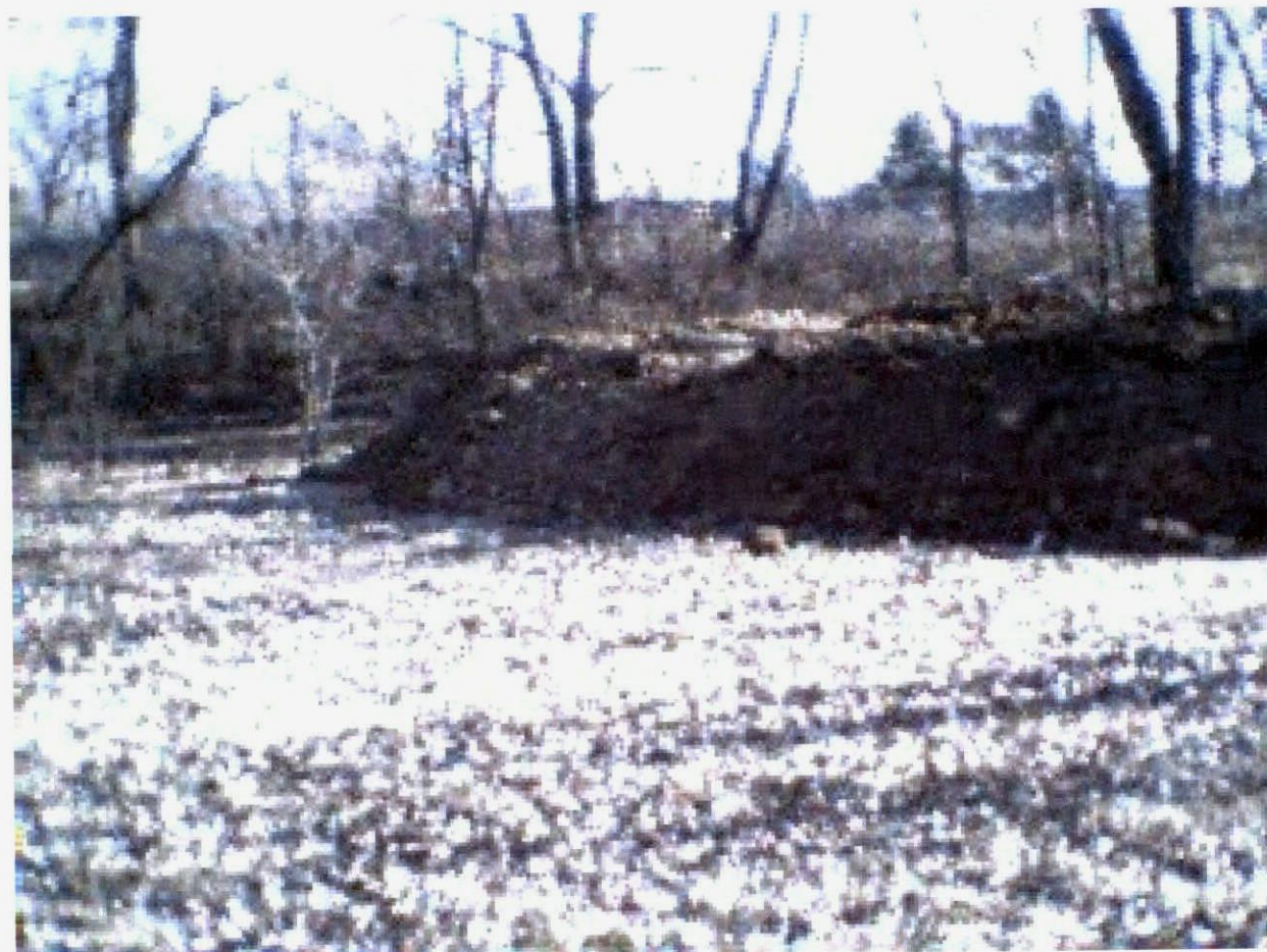
DIRT PILE LOOKING TOWARD CLOISTERS DRIVE
