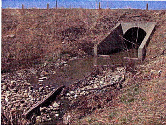
Photo #1 View of culvert under Union Pacific Railroad and drainage ditch located on the northeast portion of site.
