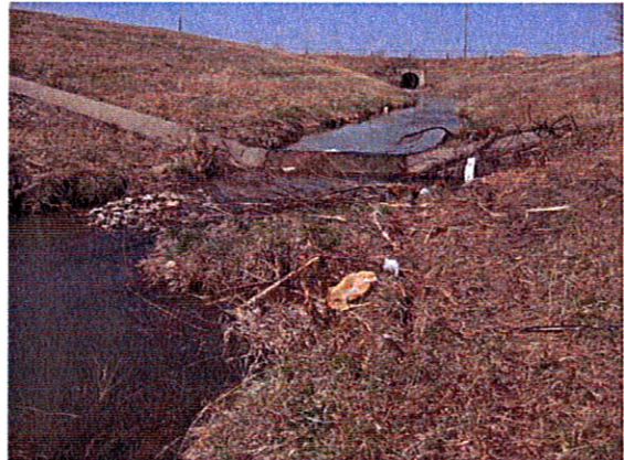
Photo #4 Looking north along drainage ditch showing check dam and location of Plot 3.
