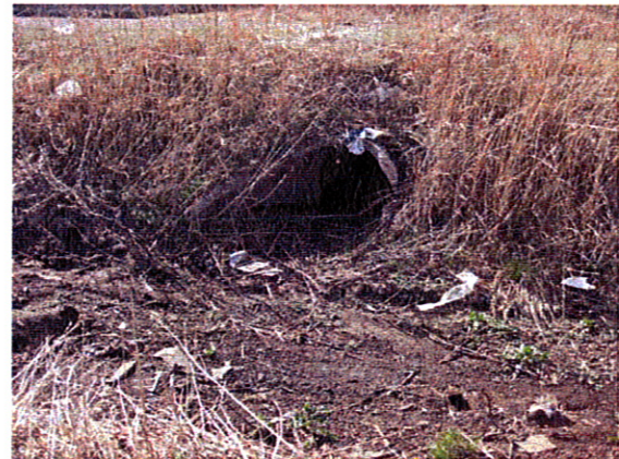
Photo #16 View of roadside ditch and culvert located on the western boundary of the site, and the location of Plot 6.
