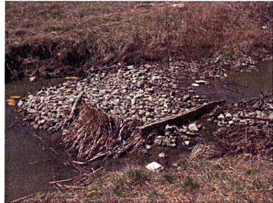
Photo #2 View of the north portion of the drainage ditch located on the site.
