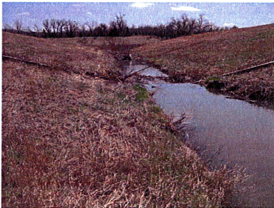
Photo #5 Looking south along drainage ditch.
