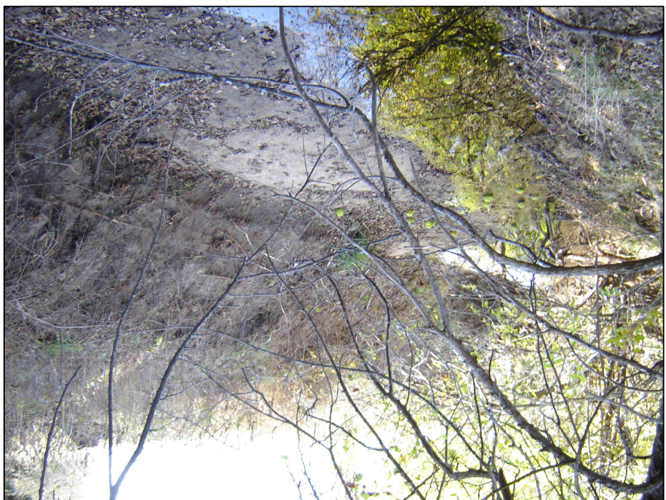
Looking east along north tributary channel (Section 30828).
