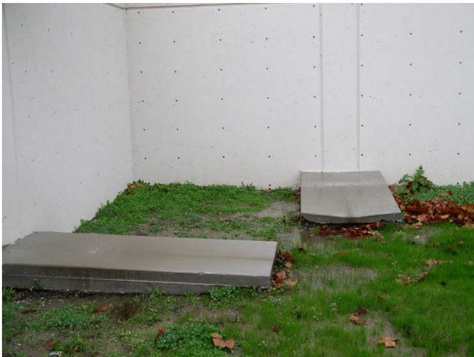
Figure 13. Scupper on east side of building.
