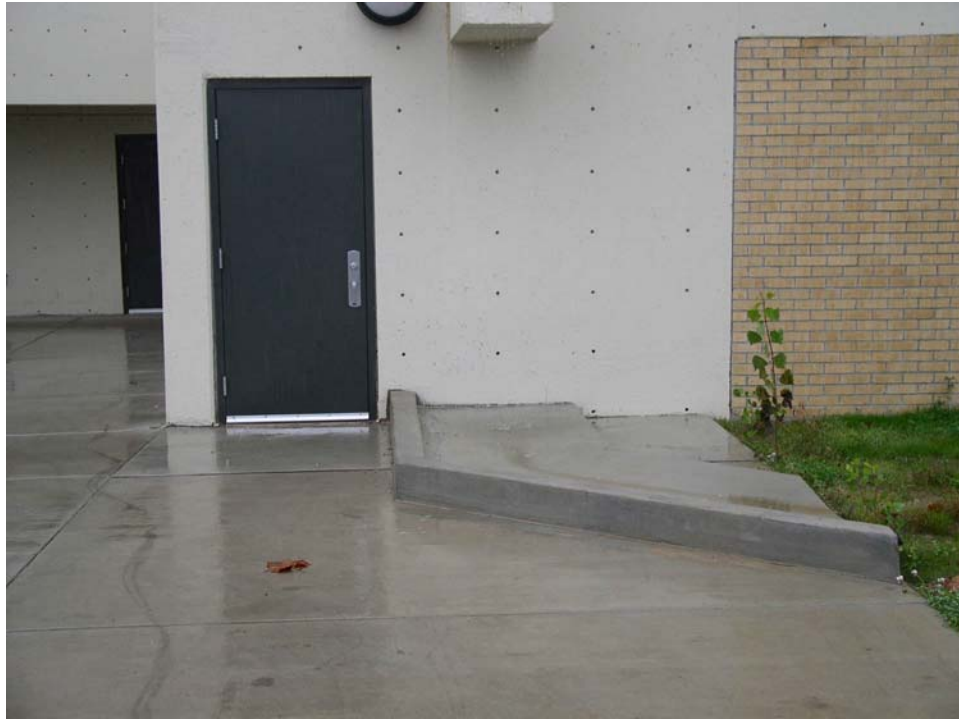
Figure 14. Door and scupper on east side of building.
