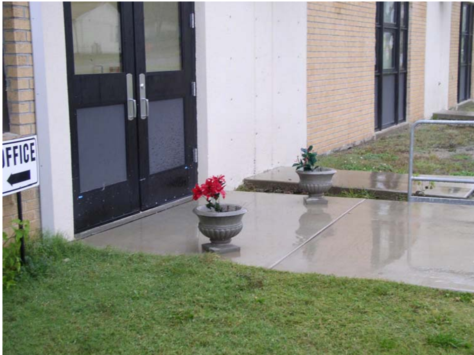
Figure 6. West door on the south side.
