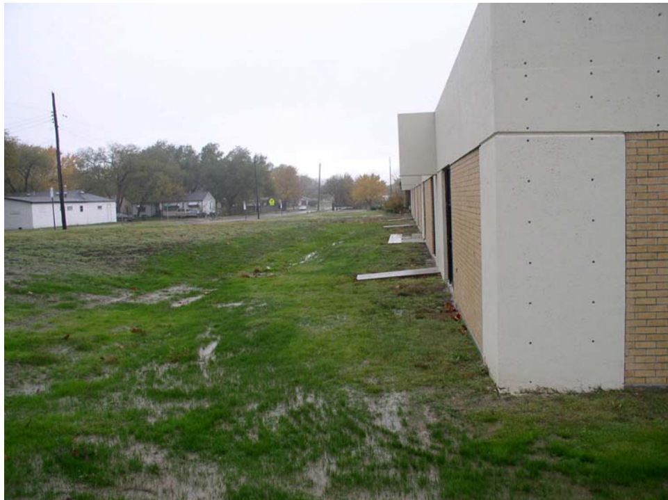
Figure 8. South side looking west.
