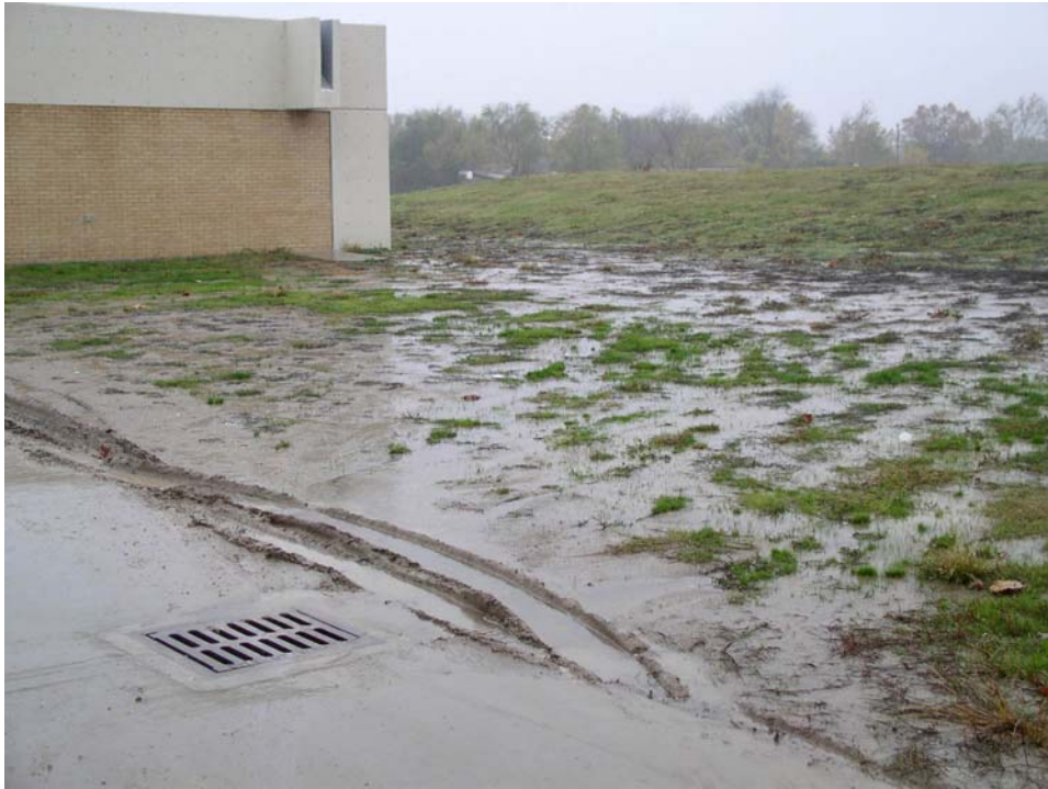
Figure 12. Inlet east of the building.
