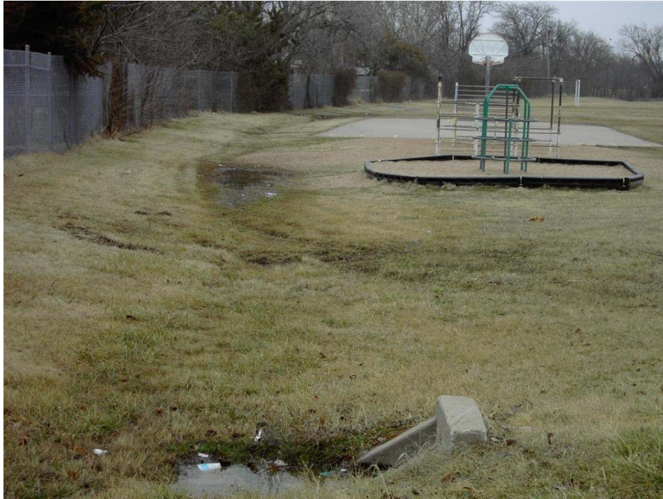
Figure 3. Swale along west property line.
