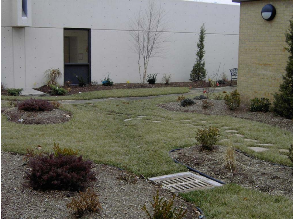
Figure 4. Inlet in the courtyard.
