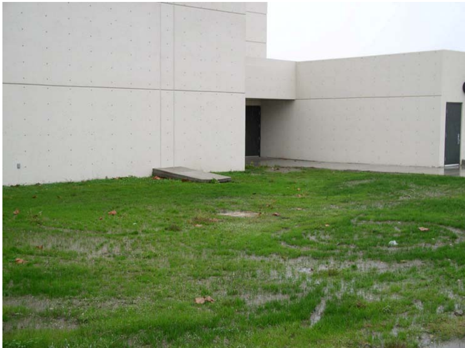
Figure 11. Inlet east of the building.
