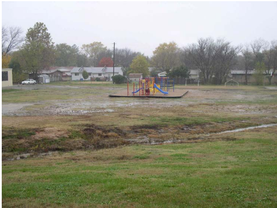
Figure 2. Water flowing across the playground.
