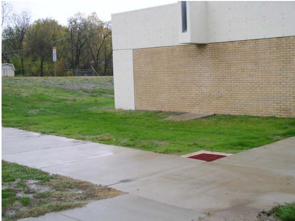
Figure 10. Inlet east of the building.
