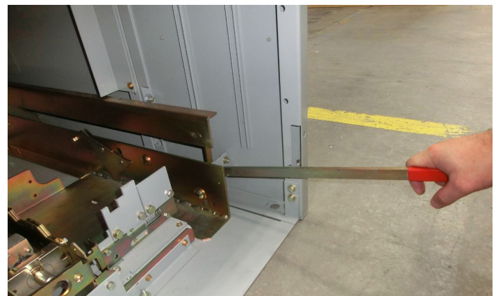
Figure 22. Hand Operation to Manually Open the Shutters
