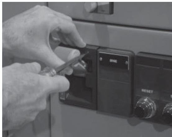
Figure 37. Defeater mechanism
