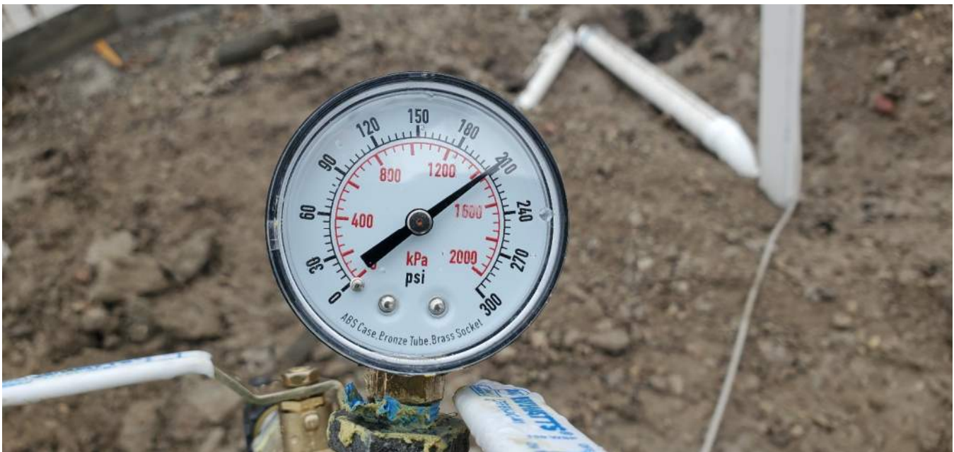
Start of hydrostatic pressure test at 10:40 AM with a pressure reading of 207 psi
