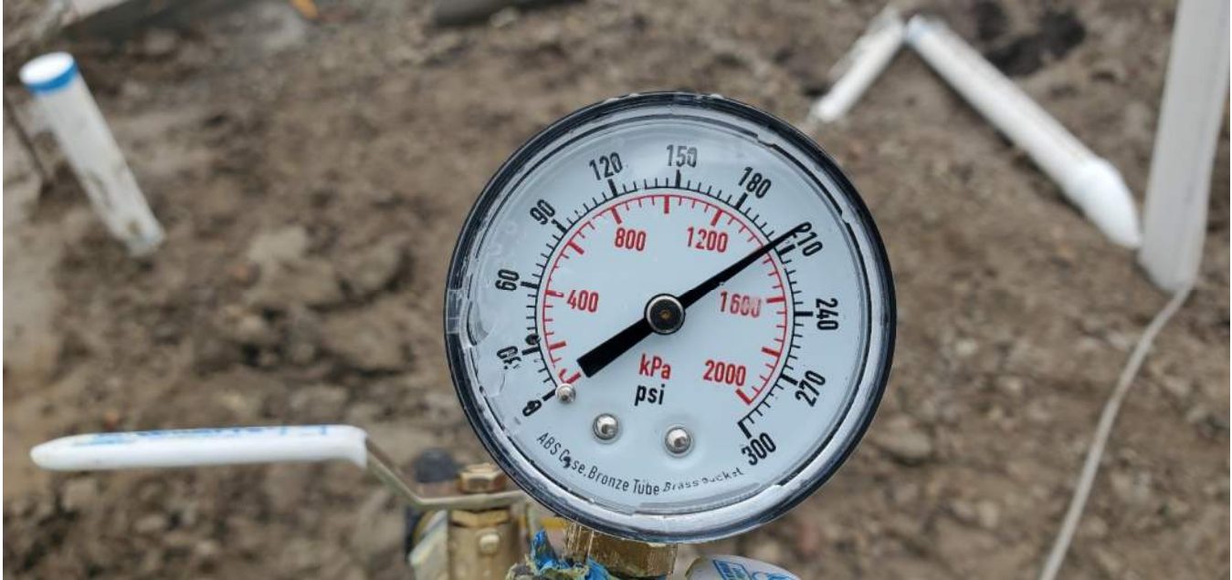
Middle of hydrostatic pressure test at 11:40 AM with a pressure reading of 205 psi
