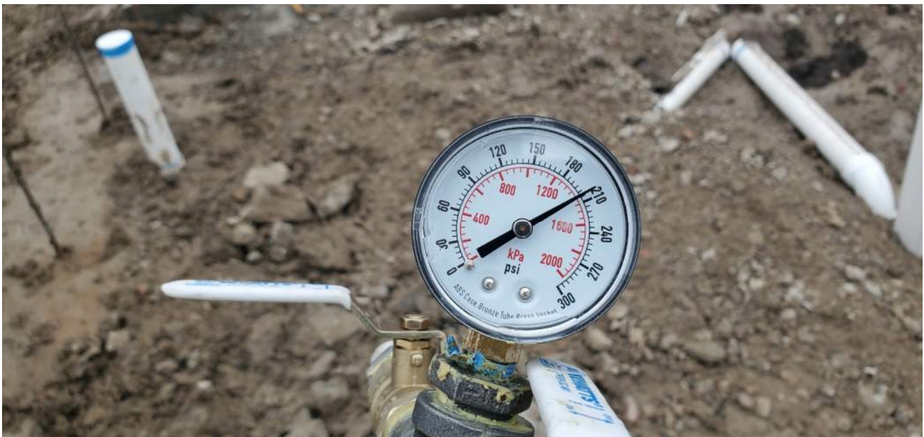
End of hydrostatic pressure test at 12:40 PM with a pressure reading of 204 psi
