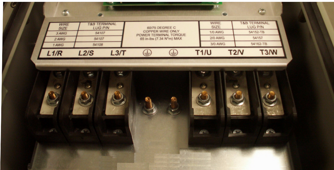
Figure 4-2: Power Terminals on Higher-HP Models
