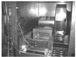
Figure 53 - 9-25 and 30 ton Supply Fan
