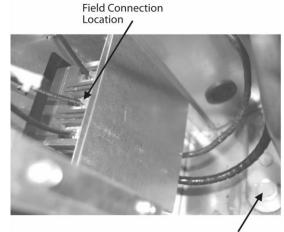
Utility Entry Figure 28 - Back View of Power Switch from Compressor and Control Compartment (6-50, 60, and 70 ton Units)
