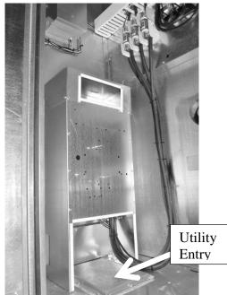
Figure 29 – Back View of Utility Entry and Power Switch from Control Compartment (55, 65 and 75-140 ton Units)
