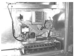
Figure 50 - Gas Heat Exchanger
