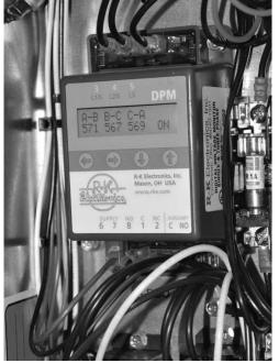
The DPM is a Digital Phase Monitor that monitors line voltages from 200VAC to 240VAC 1 $\phi$  and 200VAC to 600VAC 3 $\phi$ . The DPM is 50/60 Hz self-sensing. DPM should be wired according to unit specific wiring diagram include in the control compartment
