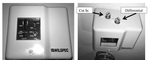
Settings for CUT IN and DIFFERENTIAL PRESSURE are indicated with two slider gauges.
