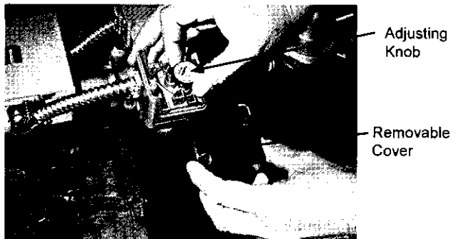
Figure E-8 Gas Pressure Switch Adjustment
