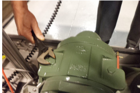
Picture 5.3.A Removing Valve Top
