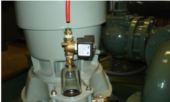
Picture 5.40 Removing the Vacuum Tubing
