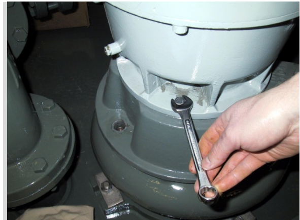
Picture 5.25 Removing Motor to Motor Adapter Capscrews
