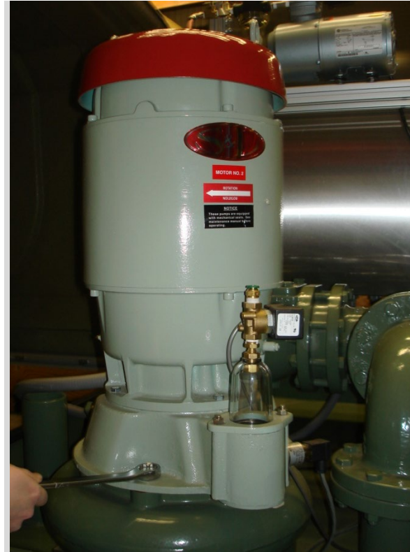
Picture 5.18 Removing Motor Adapter to Volute Capscrews
