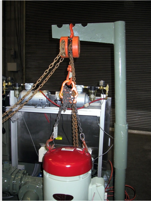
Picture 5.17 Motor Ready to Be Lifted
