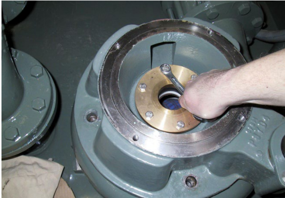
Picture 5.26 Removing Seal Housing to Motor Adapter Capscrews
