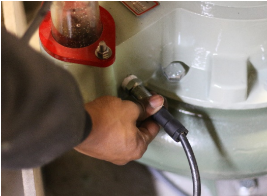
Picture 5.38 Installing WaveStart™ Cable
