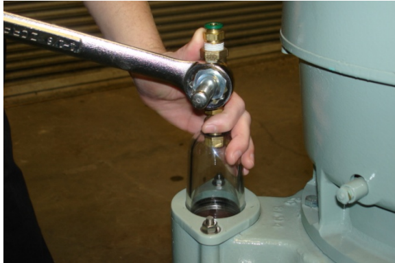
Picture 5.48 Loosening The Solenoid Valve Stem
