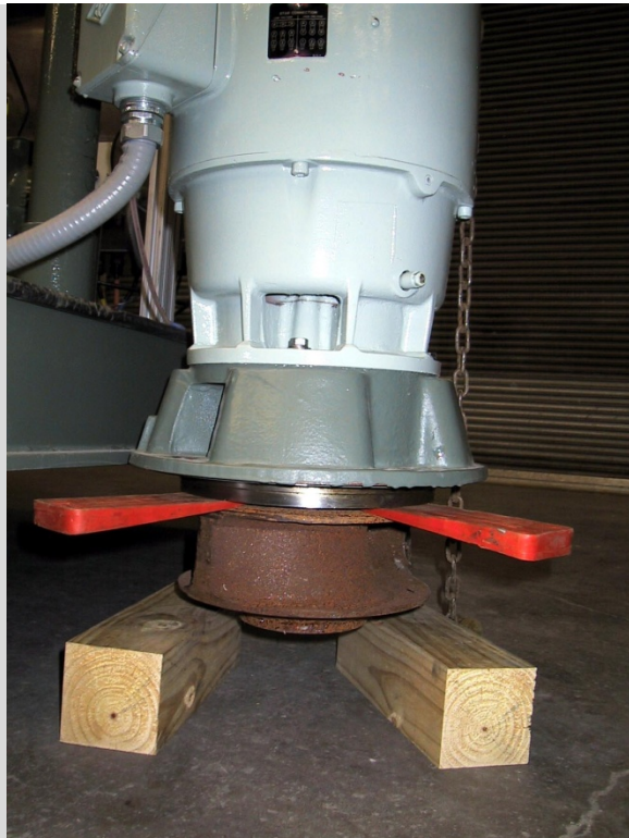
Picture 5.23 Wedges installed between impeller and motor adapter.
