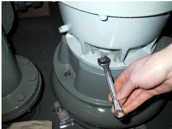
Picture 5.31 Installing Motor to Motor Adapter Capscrews
