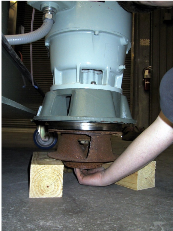
Picture 5.35 Installing New Impeller Bolt
