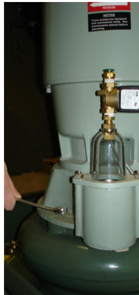
Picture 5.37 Installing Motor Adapter to Volute
