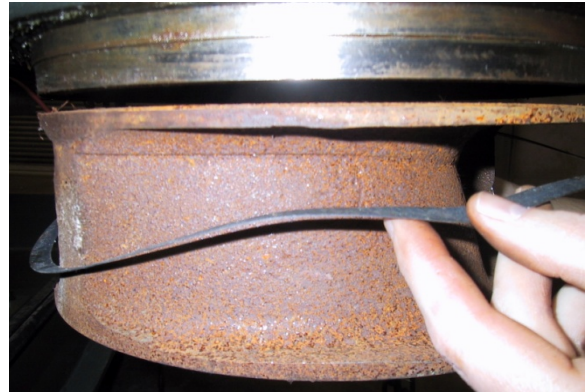
Picture 5.36 Replacing Volute Gasket
