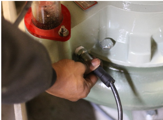
Picture 5.43 Installing the WaveStart™ Cable
