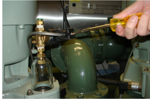
Picture 5.45 Removing Solenoid Valve DIN Connector
