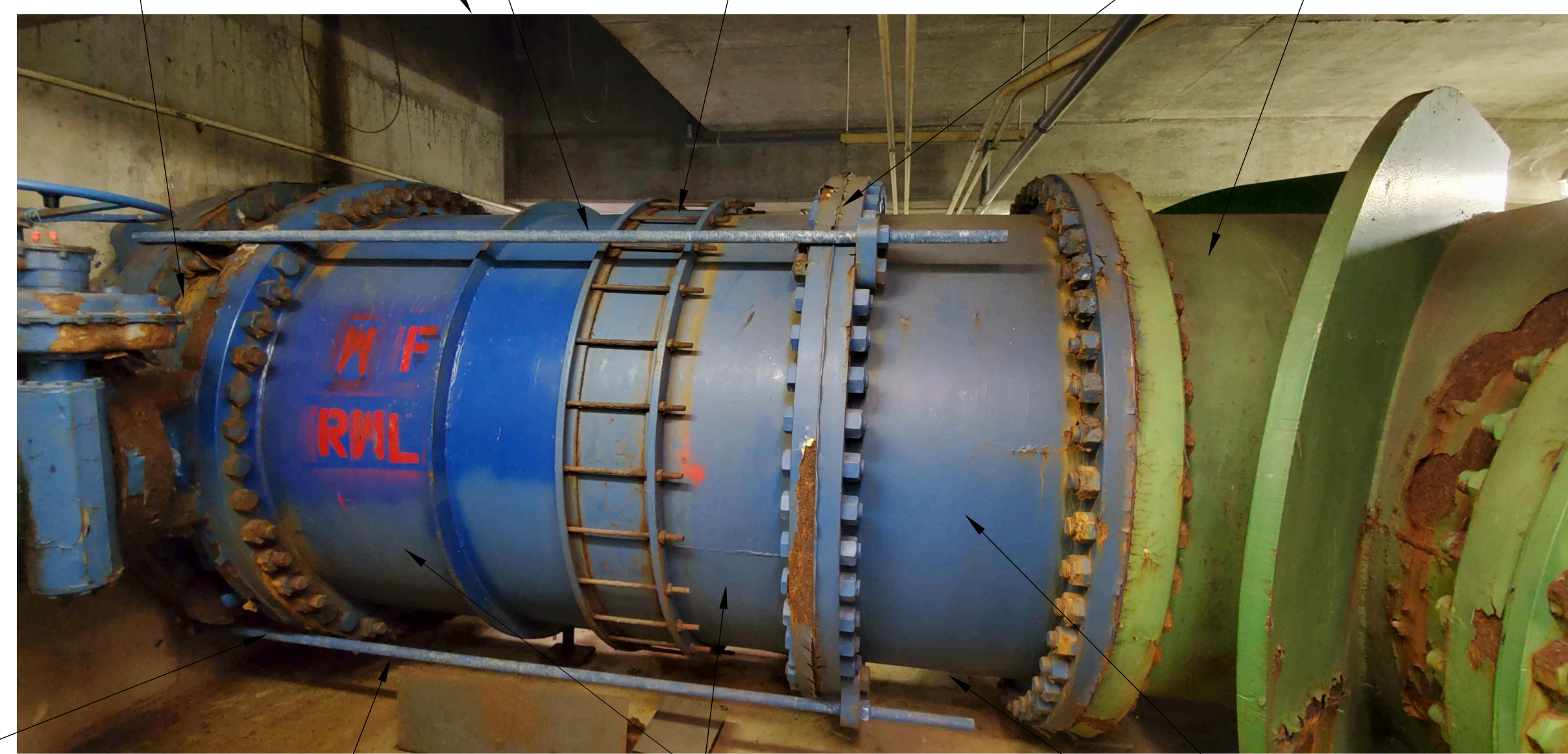
EXISTING 66" PIPE ASSEMBLY - LOOKING NORTH
