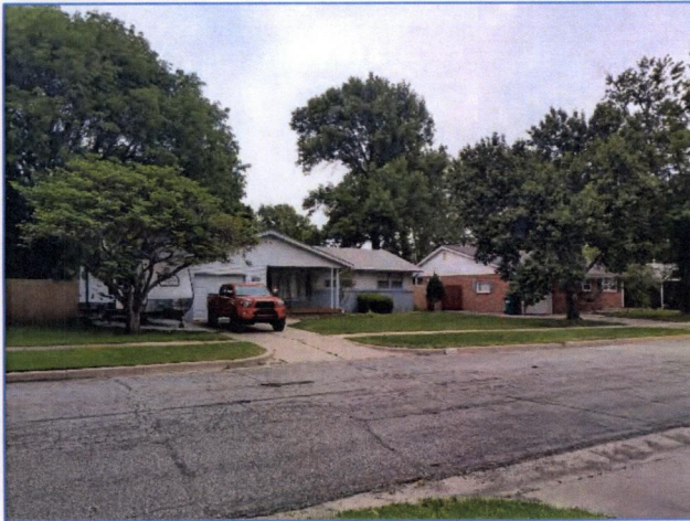
Subject Property – 2041 W. Columbine Ave.
