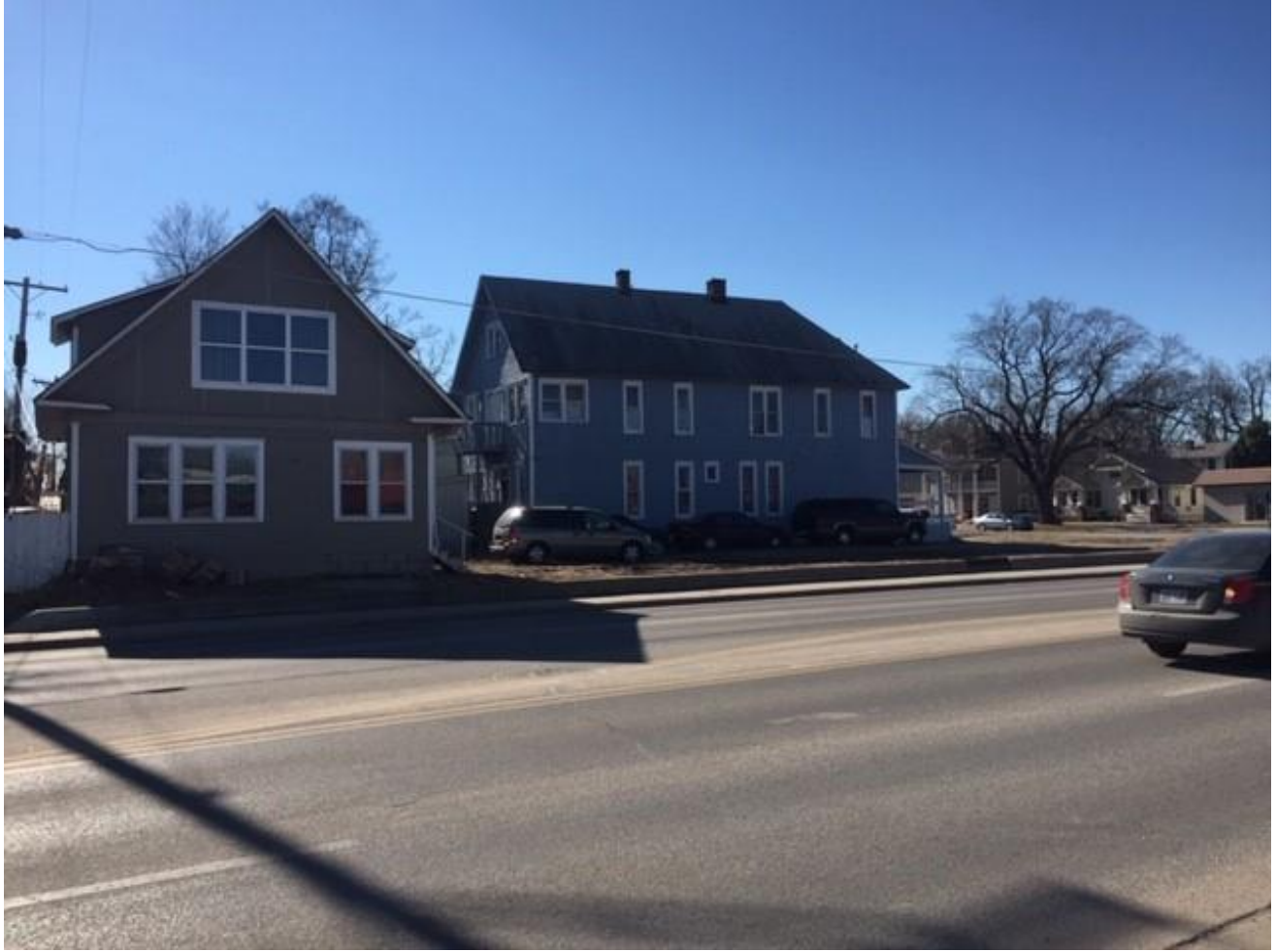
On 13th, looking south /southwest at the site
