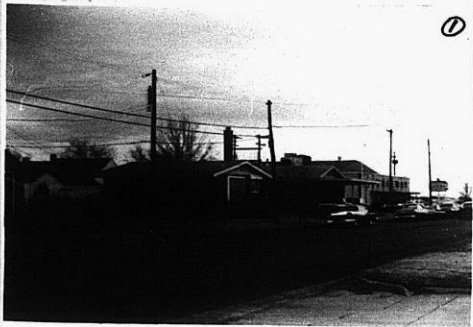
TWO OFFICES SOUTH OF APPLICATION AREA
