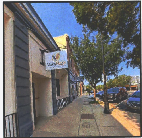
Front of 901 W. Douglas and viewing west
