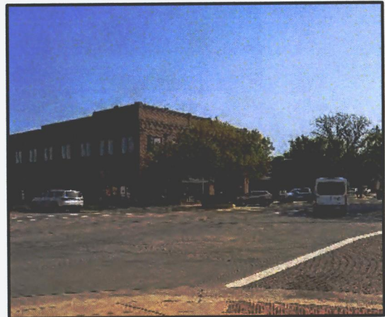
Northeast corner of Handley & Douglas -BBQ shop
