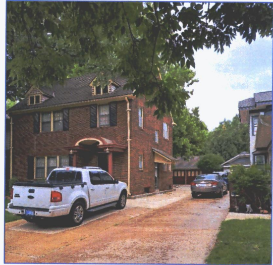
North side of subject property with apartment entrance
