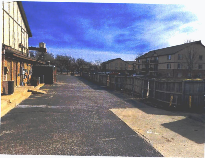
South of the subject site, facing east.
