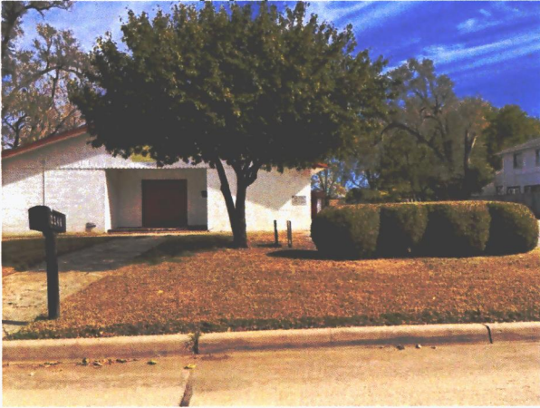
Looking east at church property
