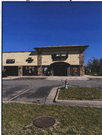
Looking north into subject site
