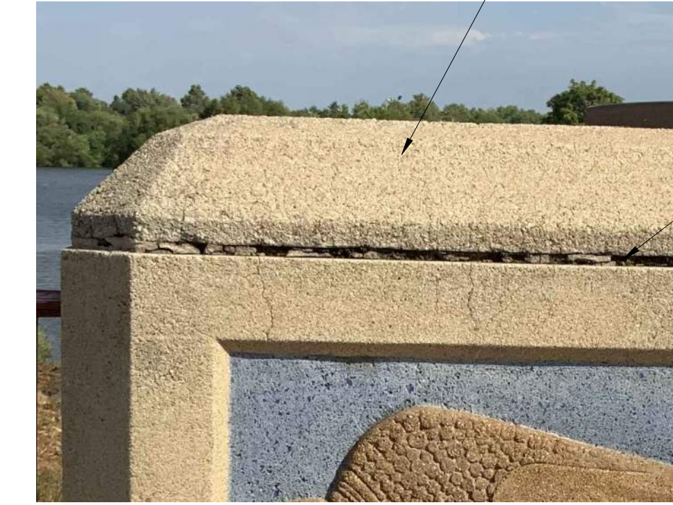
REMOVE AND REINSTALL LOOSE CAPSTONES PER 1/15
