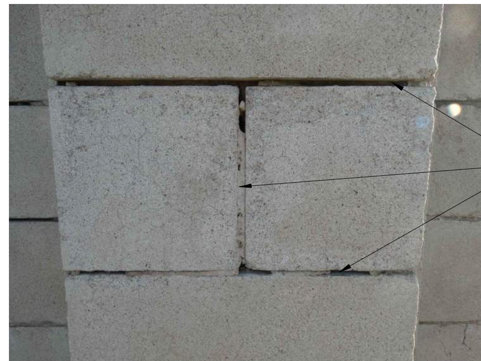
5 TYPICAL MORTAR DETERIORATION AT END WALL NOT TO SCALE
