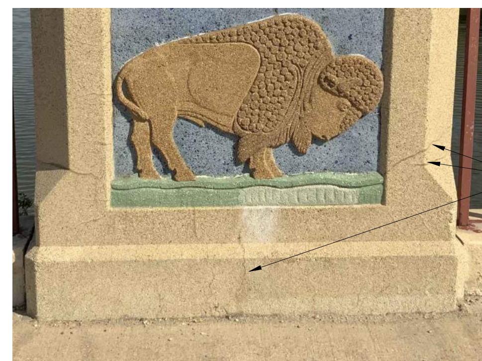
9 TYPICAL CRACKING NOT TO SCALE
