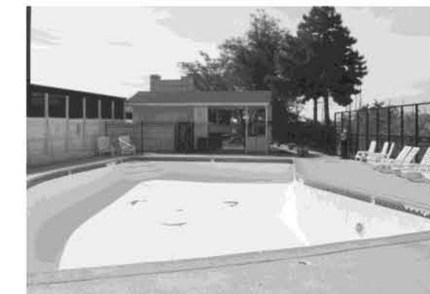
EXISTING POOL & CONCRETE DECK
