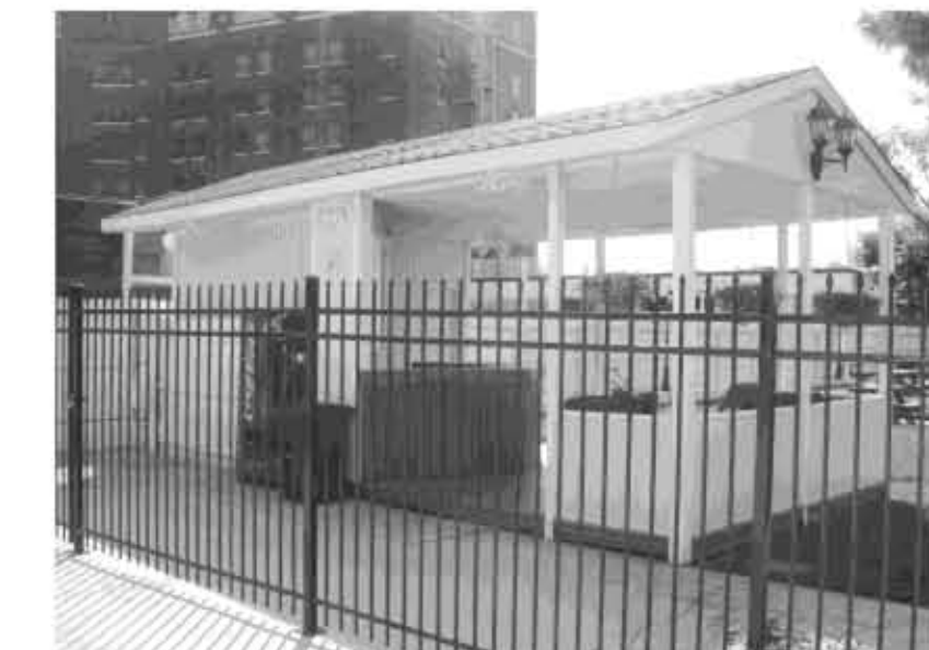
EXISTING WOOD STRUCTURE
