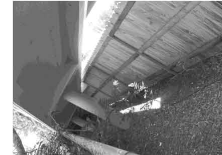
EXISTING CONCRETE RAMP & PIERS
