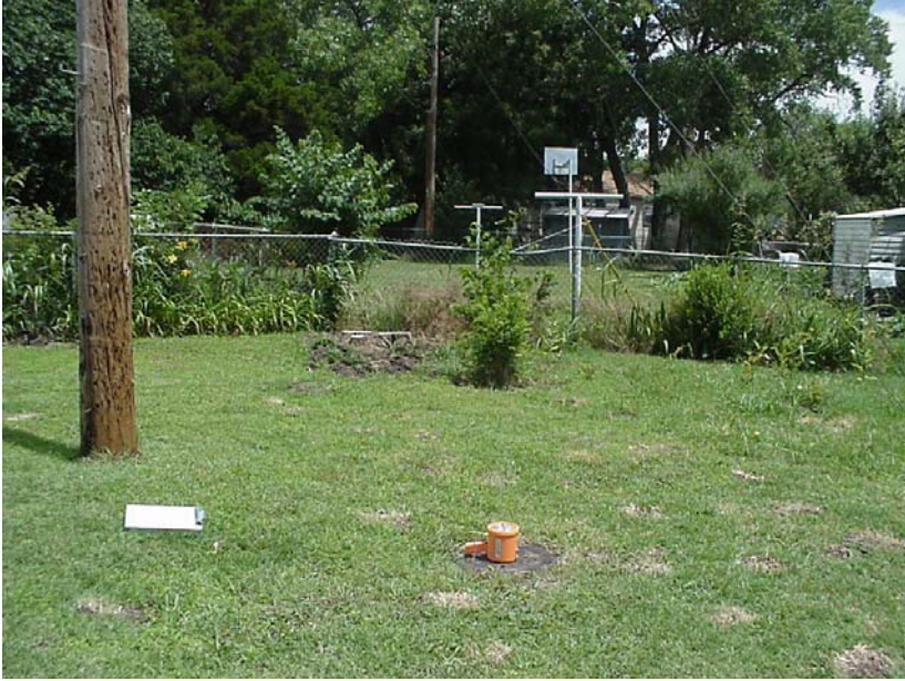
I'm standing northwest of MH 5744-793 (orange flashlight is on the manhole), looking southeast along the easement.
