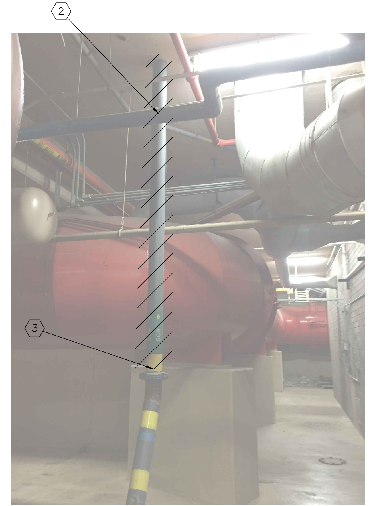
PHOTO 1- 4" SCR PIPE DEMOLITION SCALE: NOT TO SCALE
