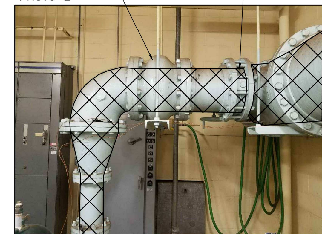
TYPICAL PUMP DISCHARGE PIPING (3 REQ'D)
