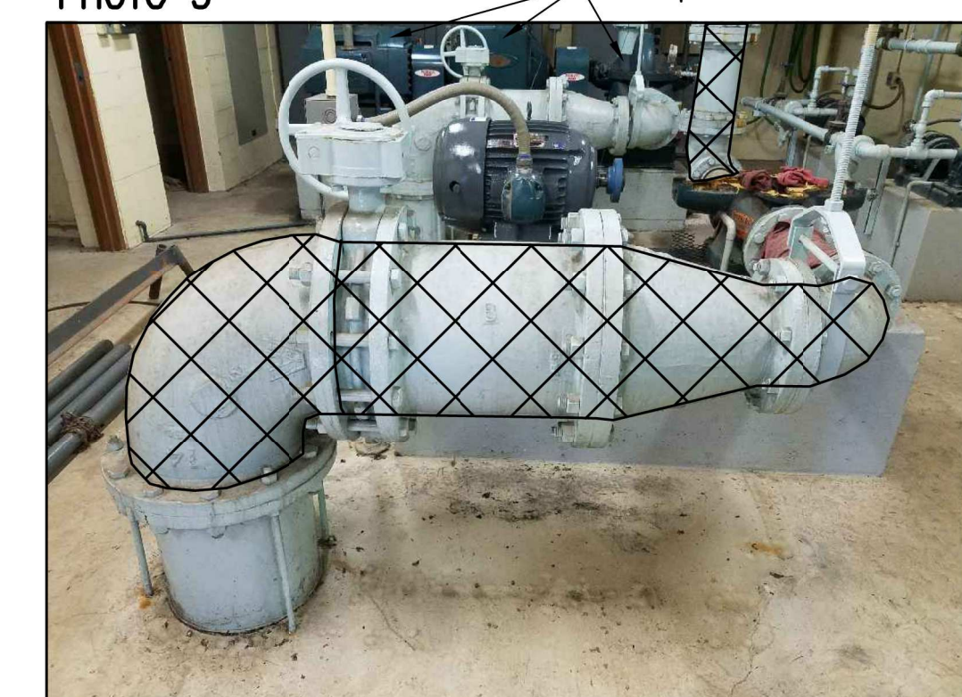
TYPICAL PUMP SUCTION PIPING (3 REQ'D)
