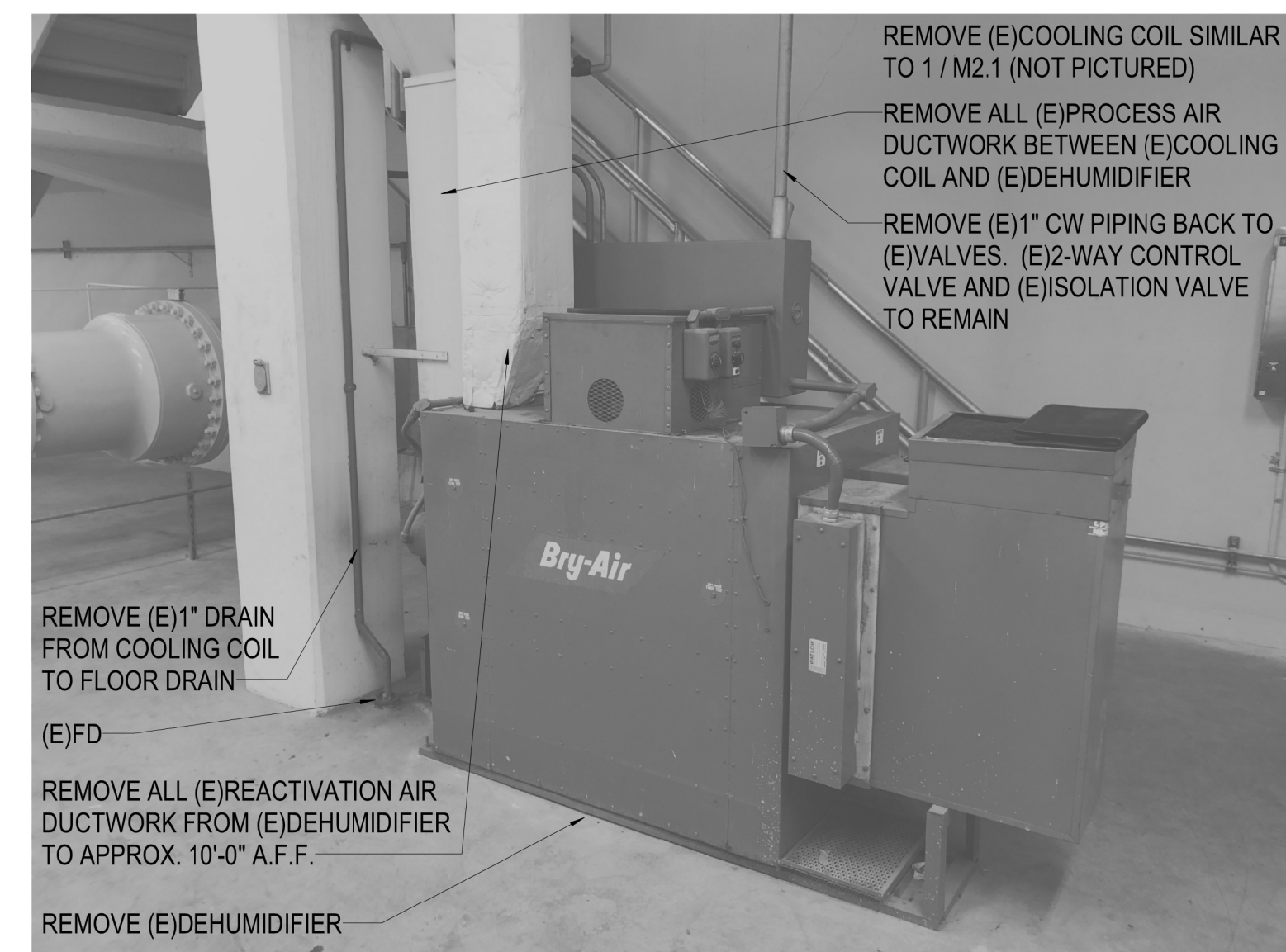
2 DEHUMIDIFIER 2 DEMO NO SCALE BASE BID
